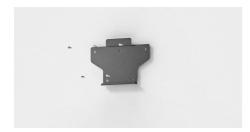
Insert the expansion tubes into the holes and tighten them, then fix the bracket onto the wall with expansion screws by using a cross screwdriver. Lift up the inverter with both hands, hang the back rail on the fixed wall bracket carefully.
